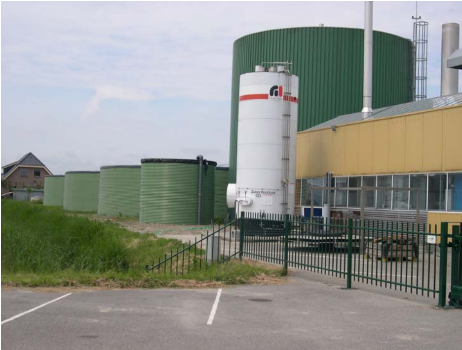
Figure 1. This property has a huge heat buffer (green), as well as a tank (white) for storage and supply of liquid ('pure') CO 2 . The smaller green tanks in the background are for water.
