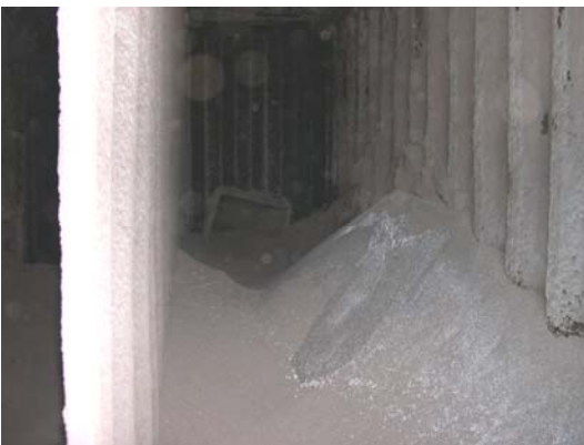
Photo 3: a look inside the first Barton Soot Collector, connected to the old boiler.
