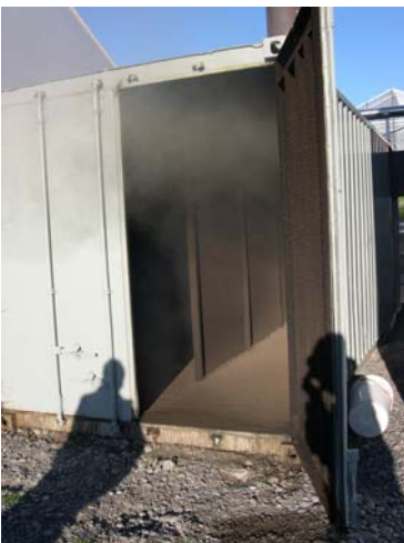
Photo 4: a look inside the new Soot Collector after 3 months.
